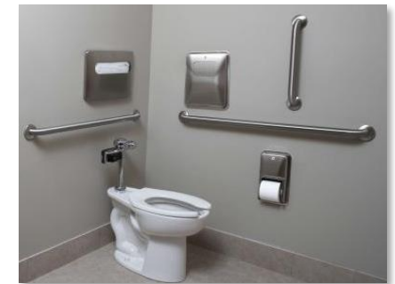
Bathroom Handrails Toilet seat and flush handle
